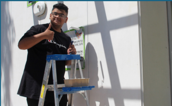
Manuel prepping wall to paint.
